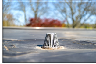
Figure 2: Roof Drain Design
