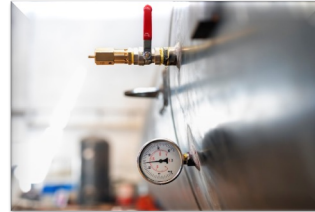
Figure 19: Pressurized tanks shall be provided with a listed pressure-relief valve
