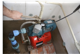
Figure 16: Potable water pumps intended to supply drinking water shall be in accordance with NSF 61
